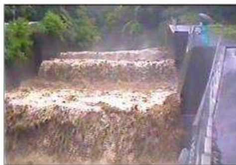
Stream intake works in flood time
